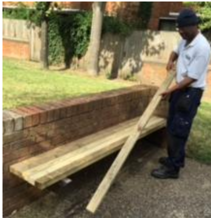
Caretaker Kelly repairing a bench by the TMO office this summer.
